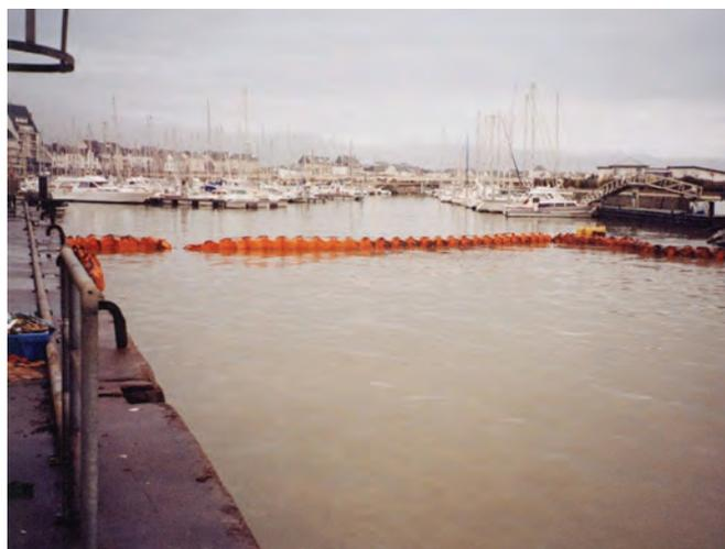
▲ *Figure 2: Successful booming of marina entrances can be compromised if the boom is damaged by vessels entering or leaving.*
