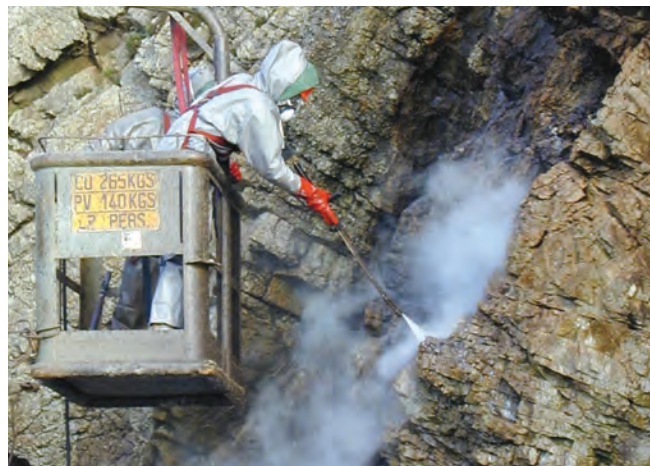
▲ Figure 21: Pressure washing a cliff face above an amenity beach. The oil was thrown high up the cliff in a storm and without cleaning would be likely to persist for some time.
