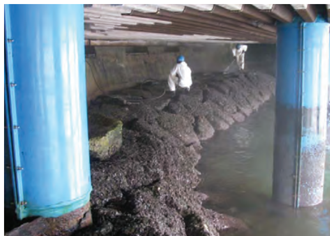
▲ Figure 31: Access underneath wharves may be difficult and dangerous for clean-up crews due to the lack of headroom and ventilation.
