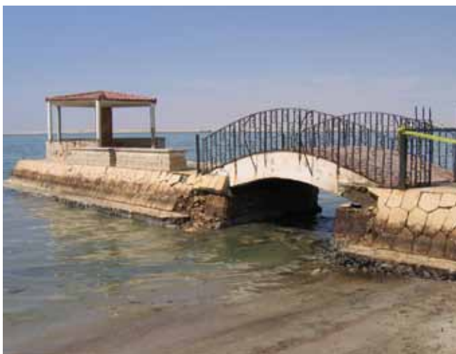
▲ Figure 14: Light oil staining of a stone jetty. This may be easily confused with algae growth.
