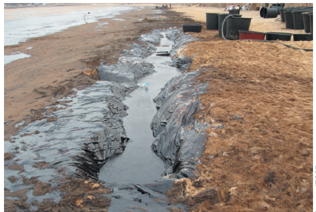
Use of a trench to recover oil
