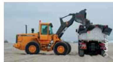
Truck and skip protected with plastic liner
