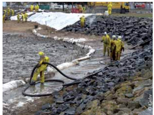
Mechanical clean-up of riprap
