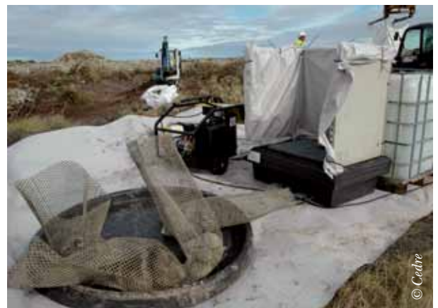
Washing pebbles on site in a booth
