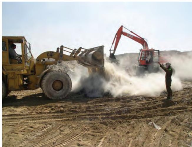
▲ *Figure 18: Stabilisation of oily waste using quicklime.*
